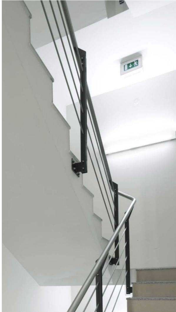
Given that corridors and stairways fulfill the role of escape routes, it is necessary, when planning, to count on the installation of emergency and safety luminaires in accordance with current standards (see the chapter 'Emergency and safety lighting').
