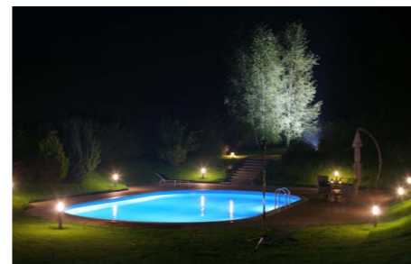
Bollards are ideal for the illumination of outdoor pools, acting to provide both sufficient light levels as well as to guide guests towards the pool, doors and amenities. Such lighting will continue the horizontal illumination from the pool into the surrounding area. For outdoor application, luminaires must have a minimum protection rating of IP 54.
