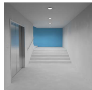
Corridors and stairways are also emergency routes in the case of an unexpected event. It is therefore a legal requirement to provide suitable emergency lighting in these areas.
