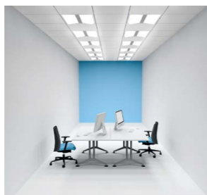
Another good luminaire choice would be recessed luminaires with specially adjusted diffusers enabling both direct and indirect light distribution that ensures sufficient illuminance of the walls and ceiling.
